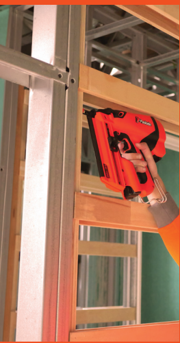
Steel Frame Fix out
